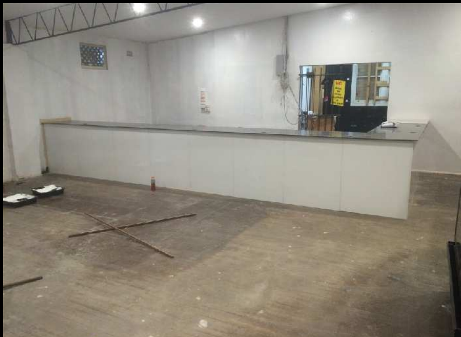
Tennis clubhouse renovation 2014
